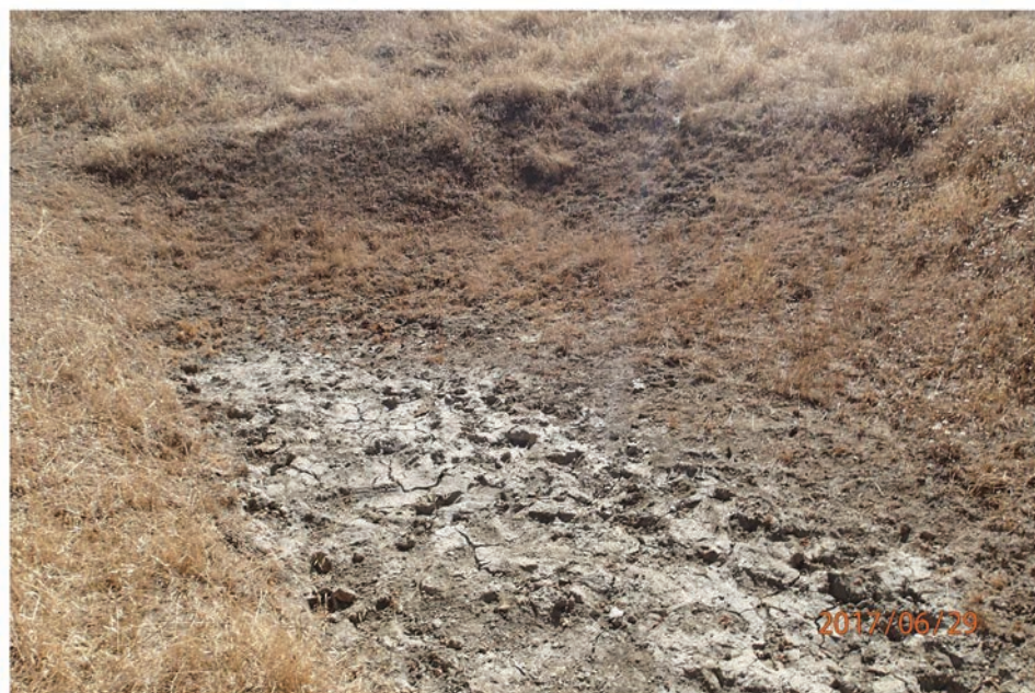
4 View From Dam.JPG
