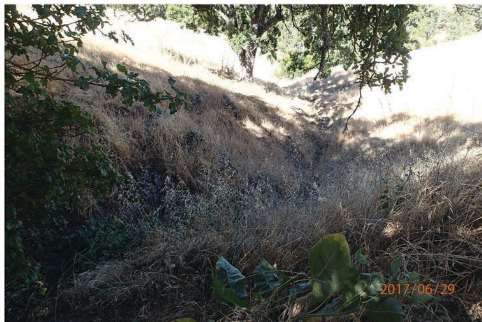
5C Facing Downstream.JPG
