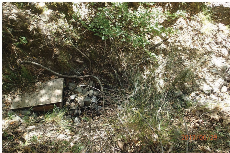
7 Downstream of Springbox.JPG
