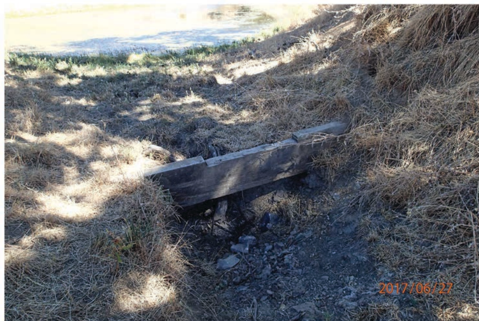
2 Downstream of Spillway.JPG
