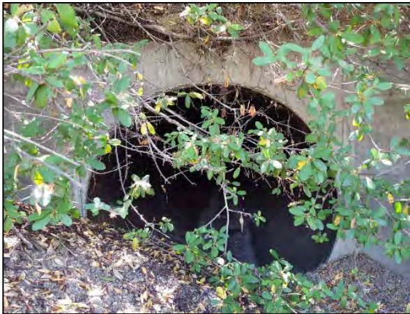
Photo 3. Culvert under Highway 101 at linkage number 10.
