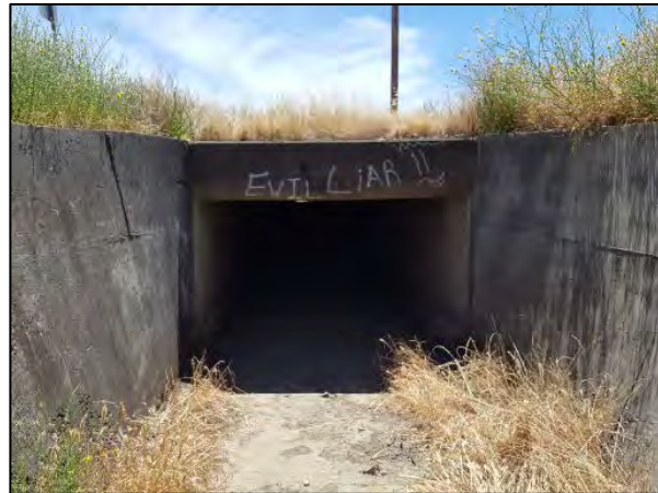
Photo 4. Culvert under Highway 101 at linkage number 11.
