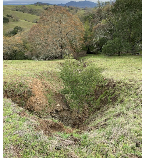
Figure 3. Pond RC-10 – (L-R) Looking down from the Access Road, Eroded Gully at Spillway
